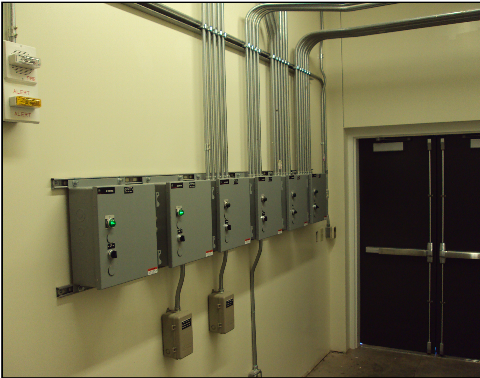
Lighting Contactors – Controls Site and Interior Lights
