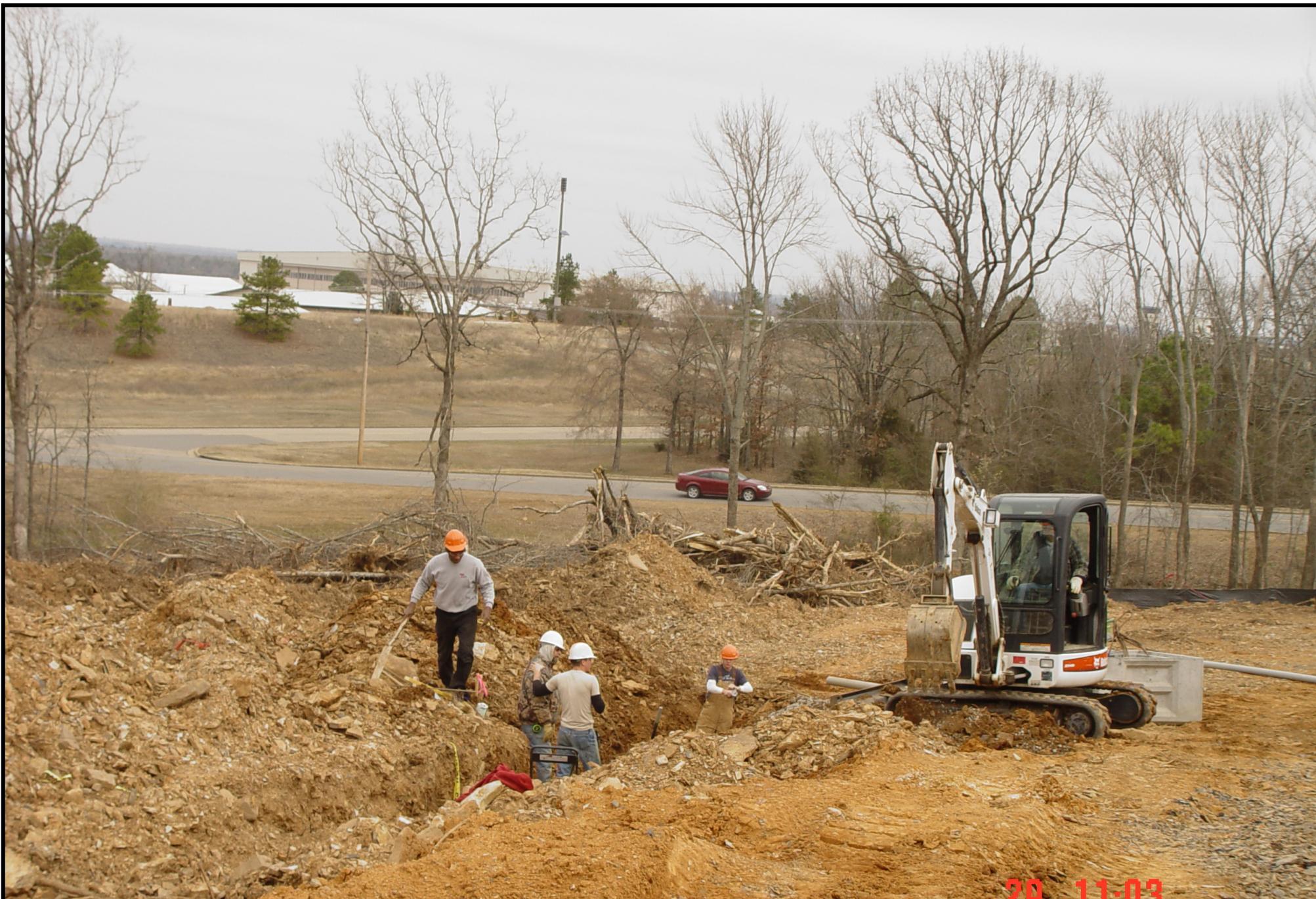
Installation of Underground Electrical Duct Bank
