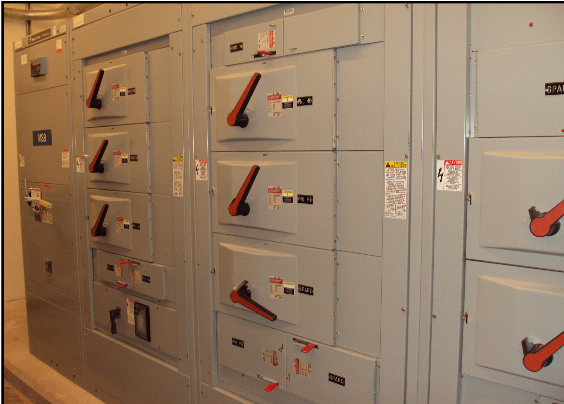
Main Switchgear – 2400 Amp, 4 sections
