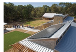
The Aldo Leopold Legacy Center's roof-mounted solar array is projected to meet 110 percent of the building's energy needs on an annual basis.
