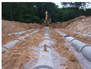
H&H Group Inc. approached its Aldo Leopold Center net-zero-energy project using a number of strategies, including an air chamber forced air system (earth tubes).
