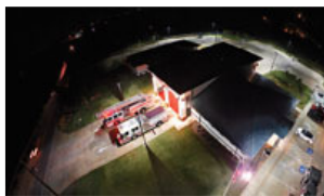
Full cutoff light fixtures illuminate the perimeter of a fire station without light trespass.
